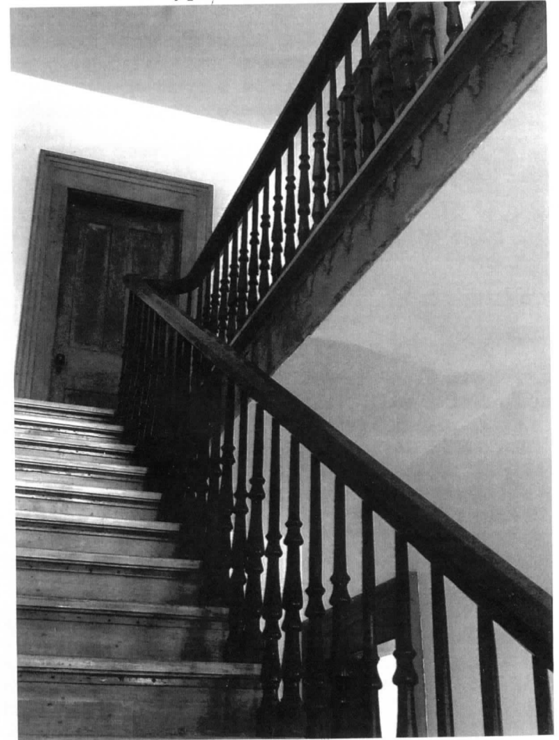
The main staircase of the Ealy House
