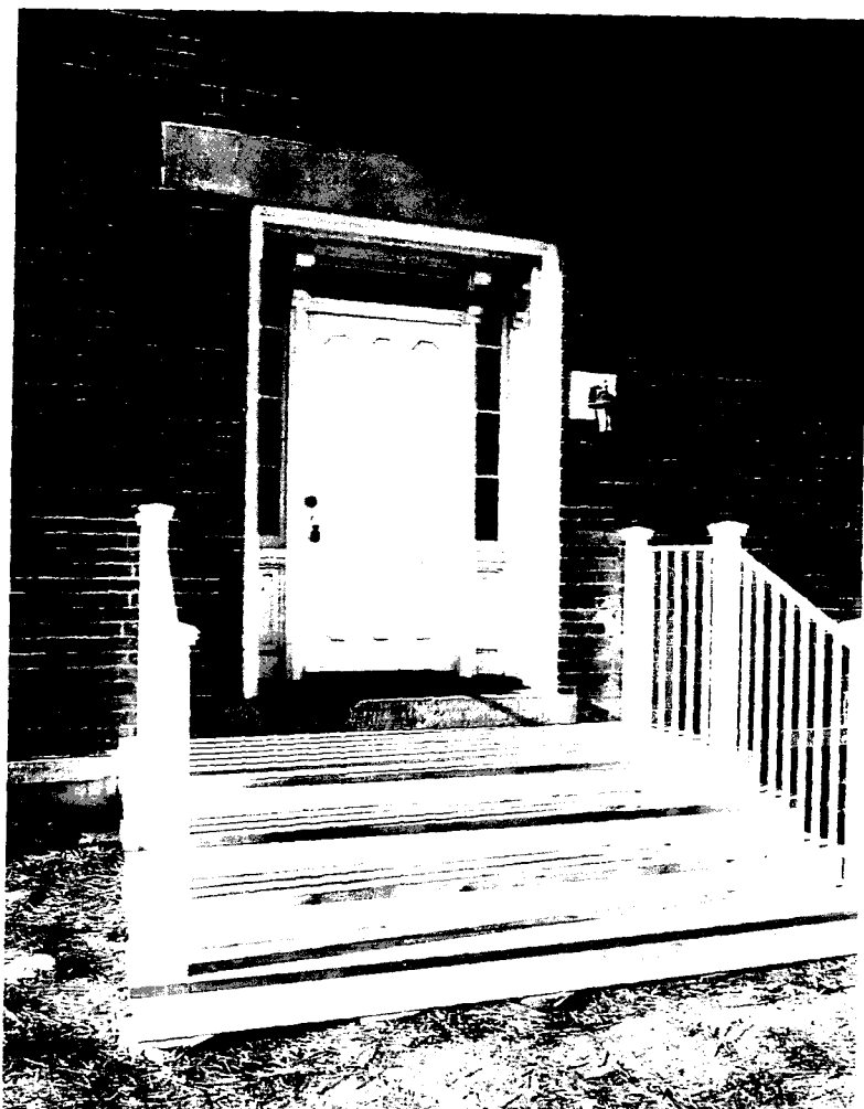
The new front steps of the Ealy House
